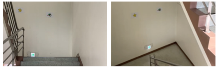
Figure 4: Image marker in staircase
